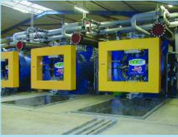
Wood impregnation plant
